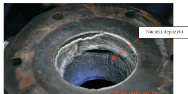
Fig. 13. Internal wall after the tests with cooled exhaust pipe (entry to the pipe) [7]
