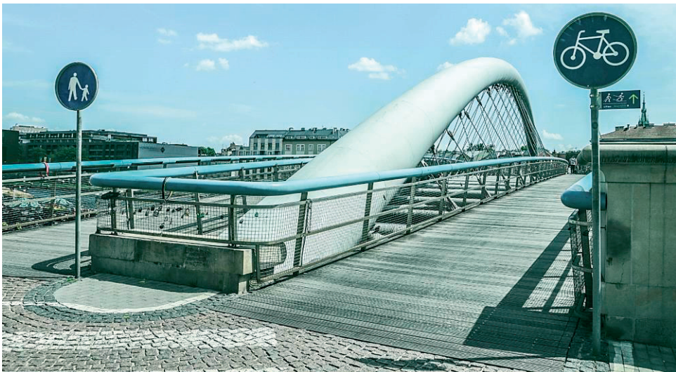
Fig. 3. Bike path on the Vistula river in Krakow (Poland) connecting the districts of Podgórze and Kazimierz. The solution completely separates bicycle traffic from pedestrians. Photo: Katarzyna Szmygin
