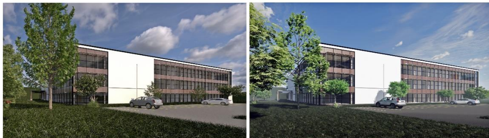
Fig. 7. Example of visualisation using different rendering techniques – Offline (V-Ray) and Real-Time (Enscape). Source: own elaboration.
