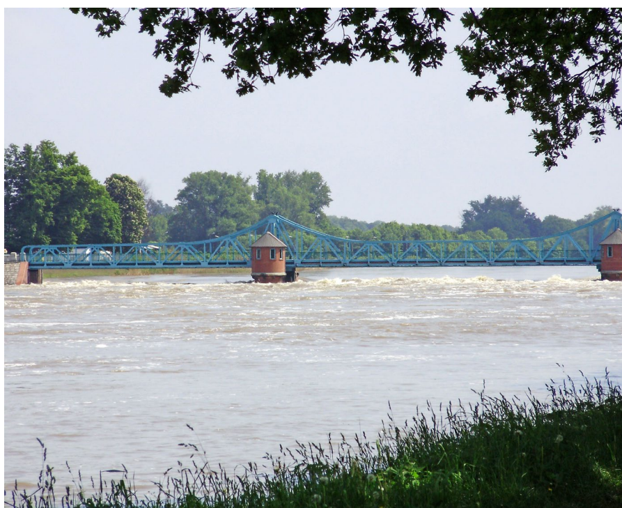
Fig. 5. Bartoszowice Weir as the main accent of layout with the surrounding plants underlines the character of the place
