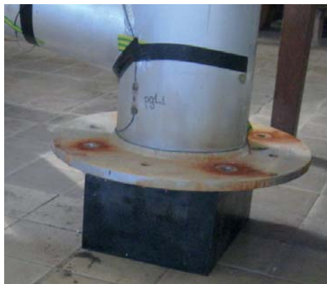
Fig. 2. Conditions of tripod foundation on rubber blocks.
