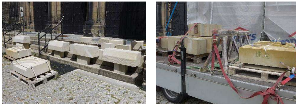
Fig. 16. New masonry units
