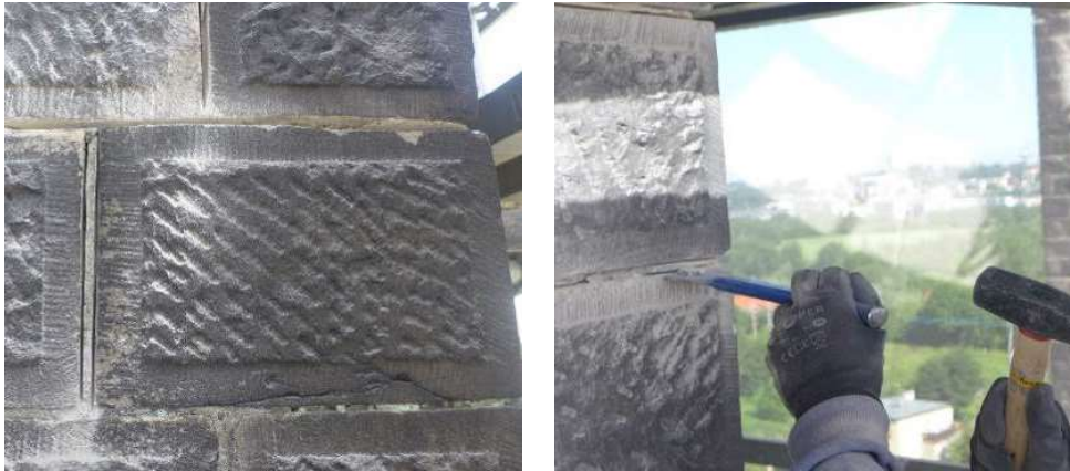
Fig. 15. Removal of secondary pointing
