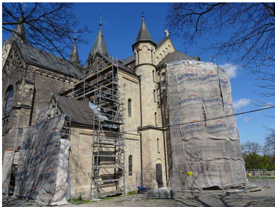
Fig. 28. Renovation of the chancel and the east elevation
