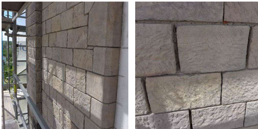
Fig. 17. Cleaned elevation and removed secondary pointing
