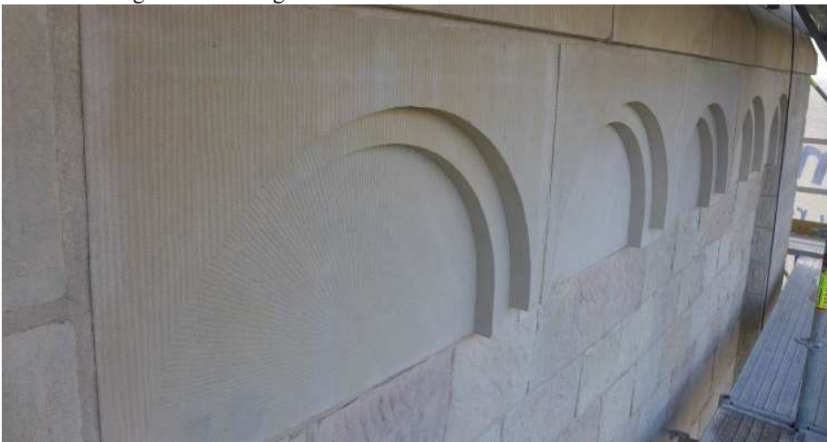
Fig. 22. Restored failure zone in the south tower
