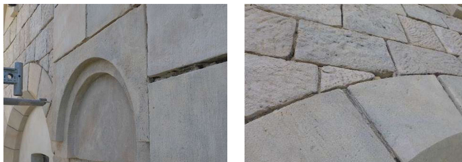
Fig. 18. Cleaned elevation and removed secondary pointing
