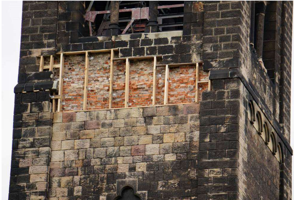
Fig. 13. Temporary protection of the debonding zone
