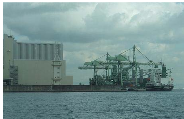
(b) Waterside warehouses
