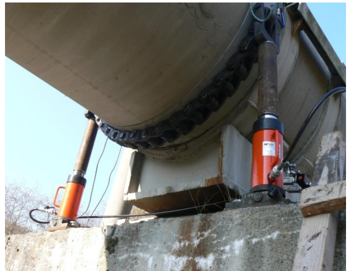
Fig. 2 Mobile lift for diagnostic and repair and restoration work on above-ground overpasses of main gas pipelines.
