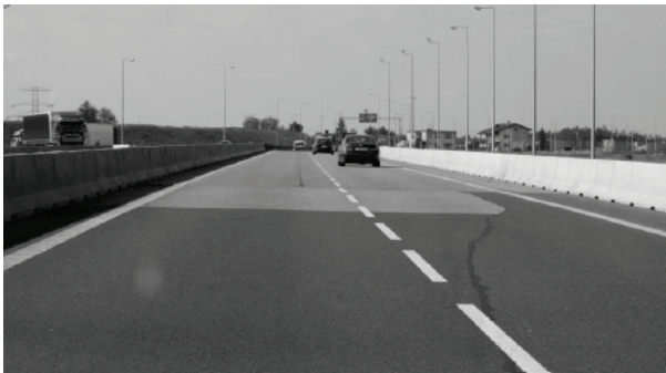
Fig. 7. Brightened asphalt pavement in Poland, A1 Belk – Świerklany [6].
