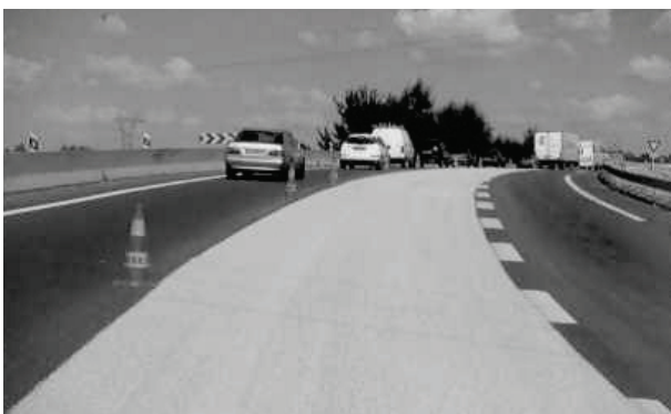
Fig. 8. Brightened asphalt pavement in Germany [6].
