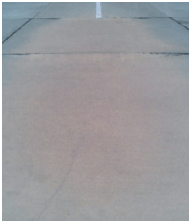
Fig. 11. Example pavement with altered colouring due to repeated impact of temperature deriving from the aircrafts' thermal emissions
