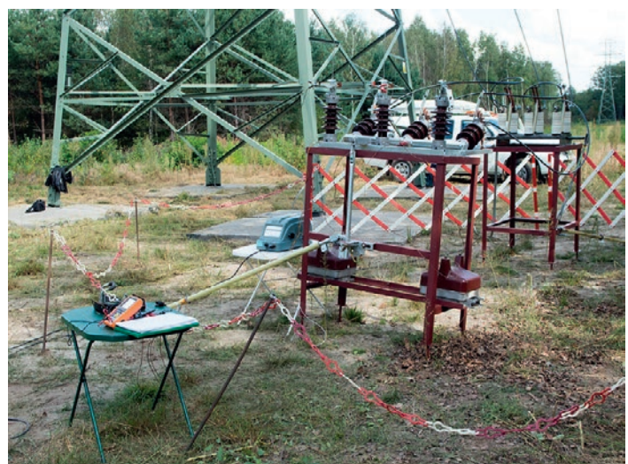
Pic. 2. Testing station used for the analysis of consequences of interactions in a four-circuit 110–15 kV line
