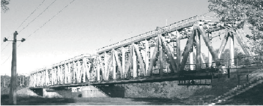
Fig. 4. Railway bridge over the Vorskla river in Poltava
