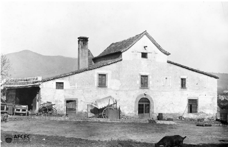
Fig. 11. Can Solà masia in Vilapicina , by the roadside of Passeig Maragall (now district VIII of Barcelona: Nou Barris ) at the beginning of the 20 th Source: AF CEC [3]
