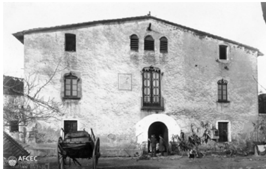
Fig. 5. Masia named Can Besora in Horta (now the district VII of Barcelona Horta-Guinardó ) at the beginning of the 20 th century. Source: AF CEC [3]
