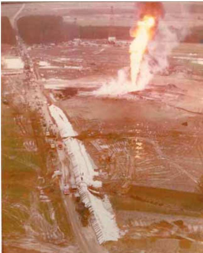
Fig. 4. General view Karlino December 1980 (source: archive of PGNIG SA in Zielona Góra)
