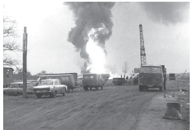
Fig. 6. Fire of oil rig December 1980 (source: Karlino Commune Office)
