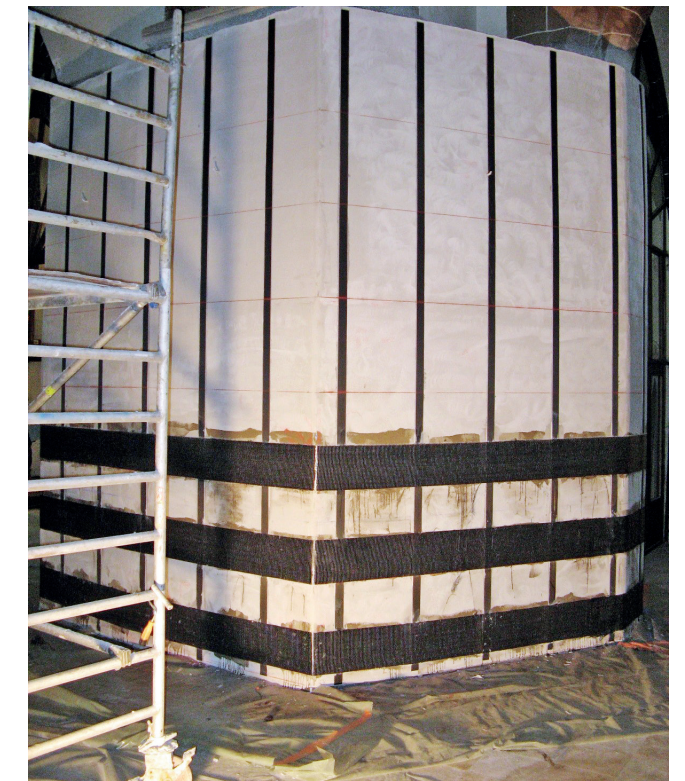
Fig. 14. CFRP-constraining strips around column base during execution
