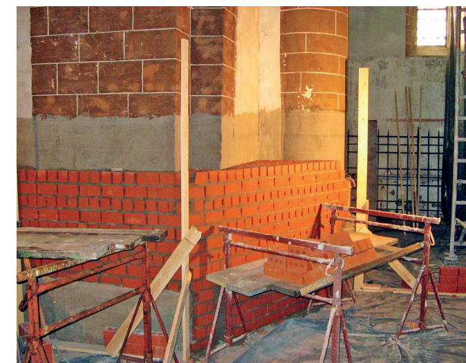
Fig. 13. Brick masonry infill in concave sections of column cross section
