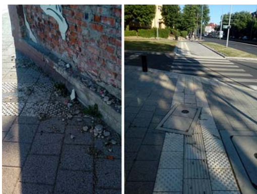
Fig. 17. Architectural barriers. Mickiewiczza street Source: the author
