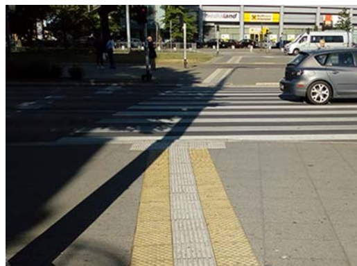
Fig. 8. Change of colors of markings in one sequence, Plac Rodła square. Source: the author
