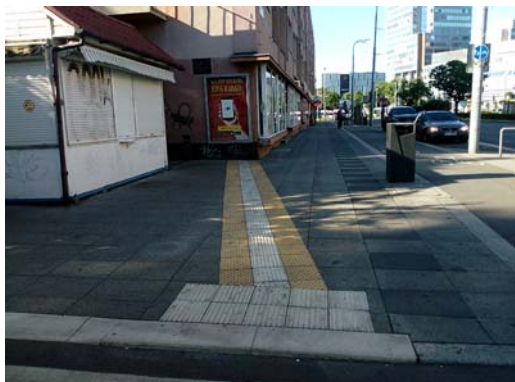
Fig. 6. Crosswalk marking for blind and visually impaired, Aleja Wyzwolenia Street. Source: the author
