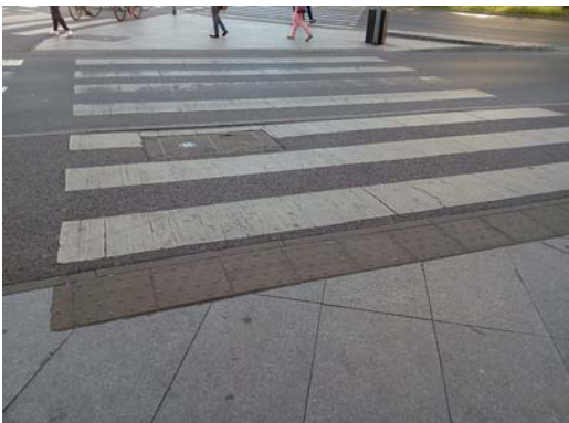
Fig. 3. Crosswalk marking for blind and visually impaired, Plac Żołnierza Polskiego square. Source: the author
