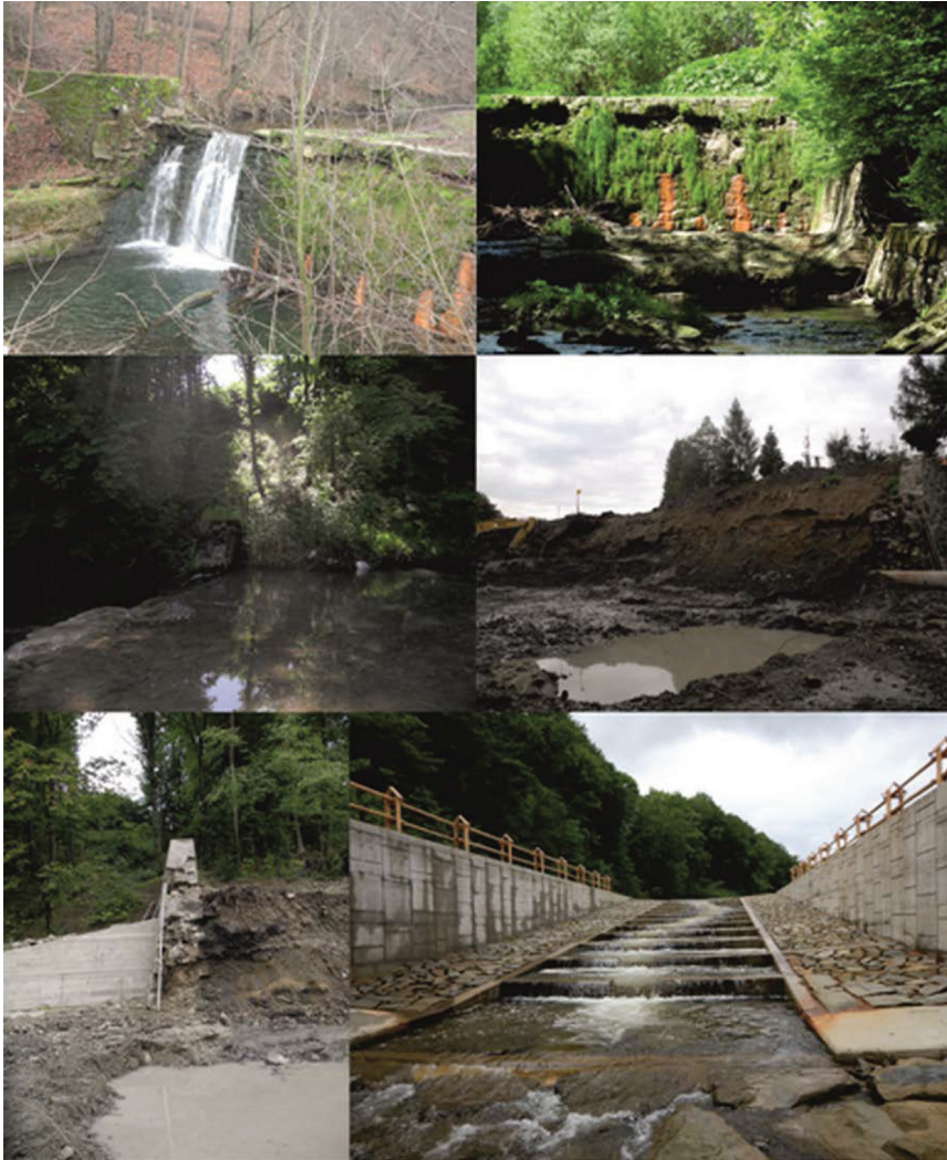
Figure 3. From the top clockwise: The dam seen from downstream – year 2012 and 2015; view upstream; reservoir after dam and deposit removal; cascade of basins in place of the main dam body; old dam remains, reservoir before the work commenced
