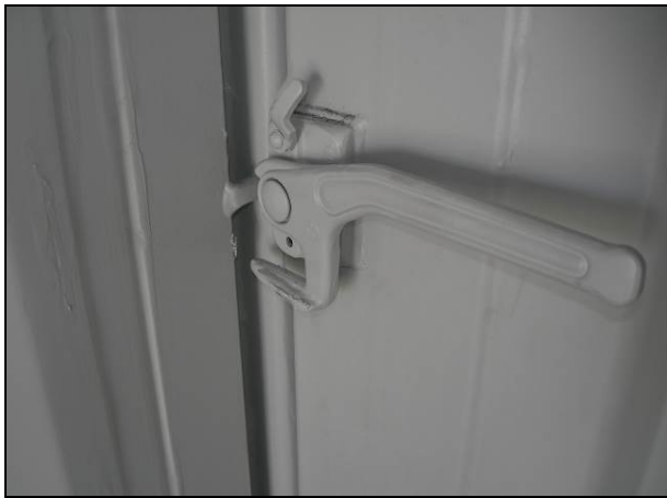
Figure 4. Bolting mechanism with handle for hinged door (from the inside).
