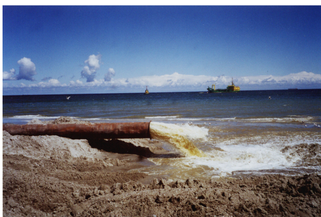
Fig. 9. The Gdynia-Orłowo beach during silting works; photo by Piotr Tatarczuk for the PRCiP
