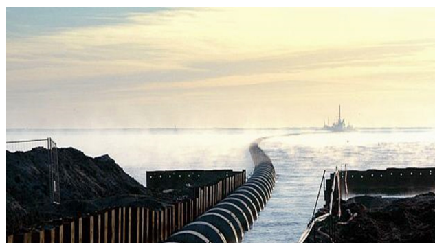
Fig. 8. A pipeline a short moment before submergence; photo by Piotr Tatarczuk for the PRCiP
