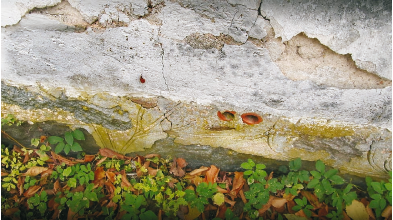
Fig. 4. A stone foundation of the house in Olszewo, its ornamented plaster and two ceramic tubes for wooden floor ventilation; source: the authors, 2021
