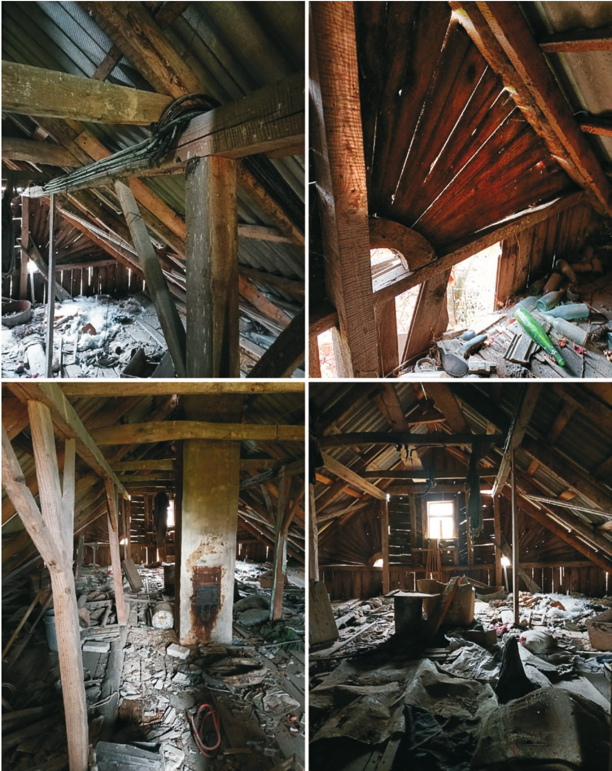
Fig. 6/a-d. A garret and roof construction; source: the authors, 2021
