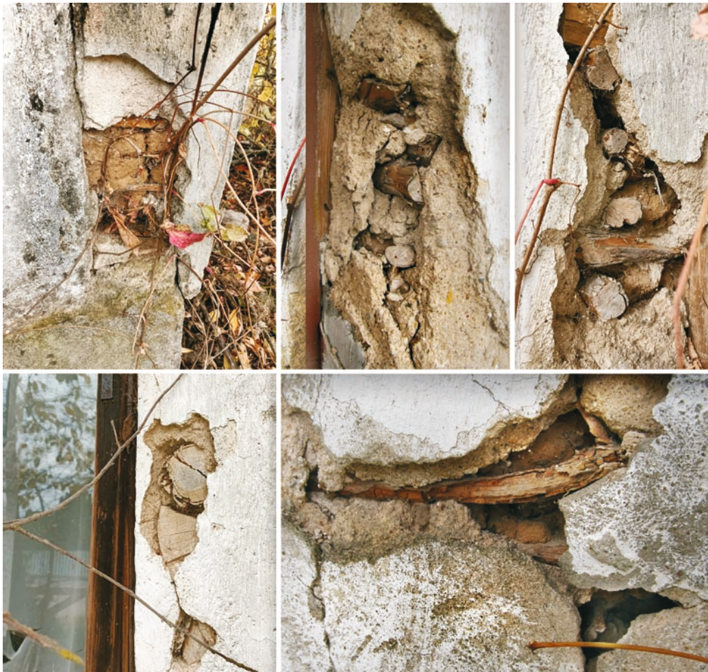
Fig. 4. A stone foundation of the house in Olszewo, its ornamented plaster and two ceramic tubes for wooden floor ventilation; source: the authors, 2021
