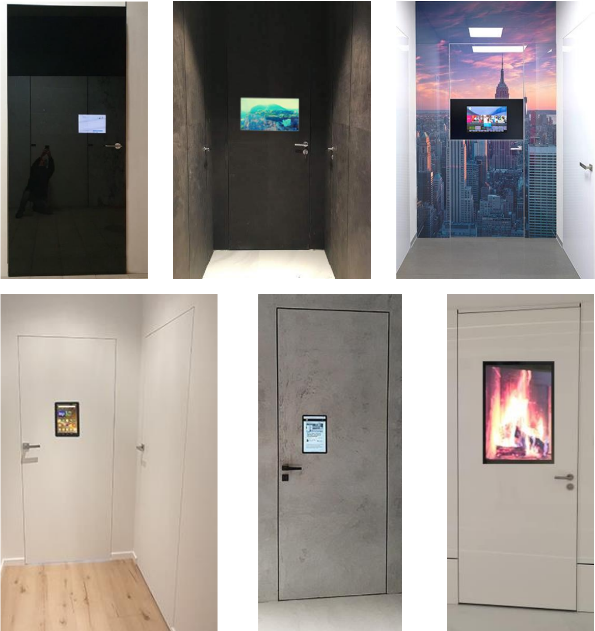
Fig. 14. Photos showing fully finished door leaf and frame assemblies with LCD monitors. Source: authors
