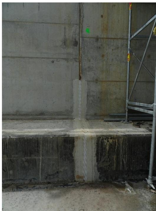
**Figure 3.** *Oblique deformation of the tape crossing the expansion joint (dilatation) of abutment P1*
