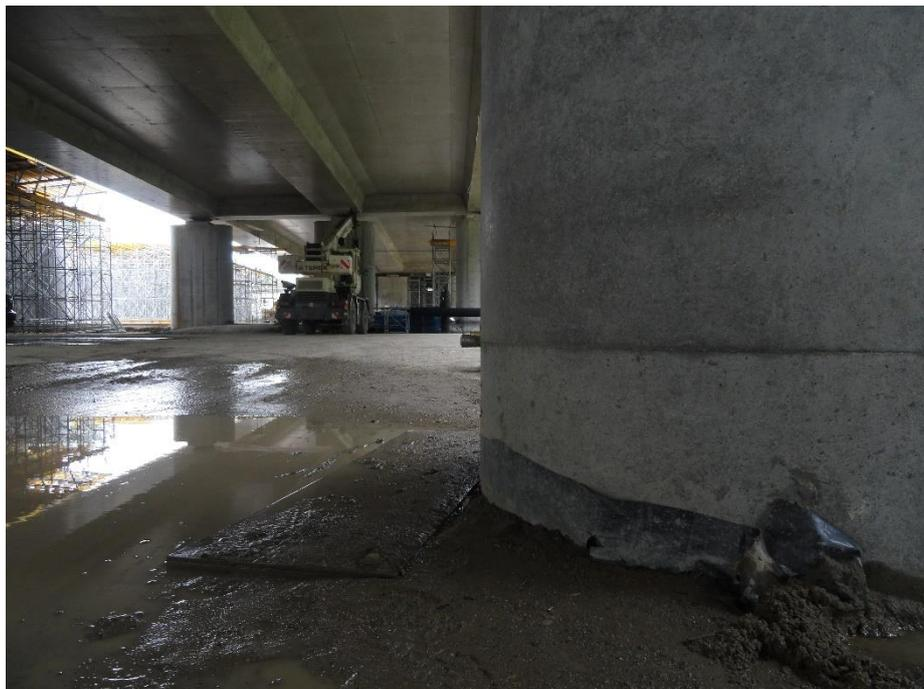
**Figure 4.** *Deformation and local depression of the working platform at support P4*
