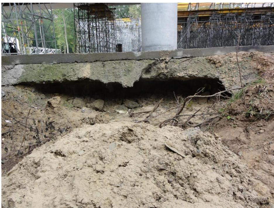
**Figure 5.** *Caverns under the working platform at support P4*
