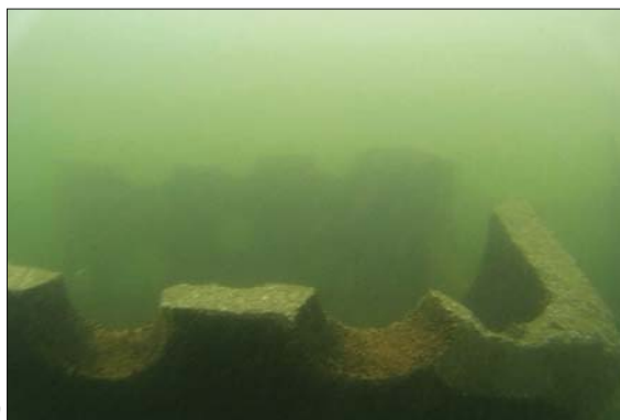
Fig. 9. Damaged elements under water
