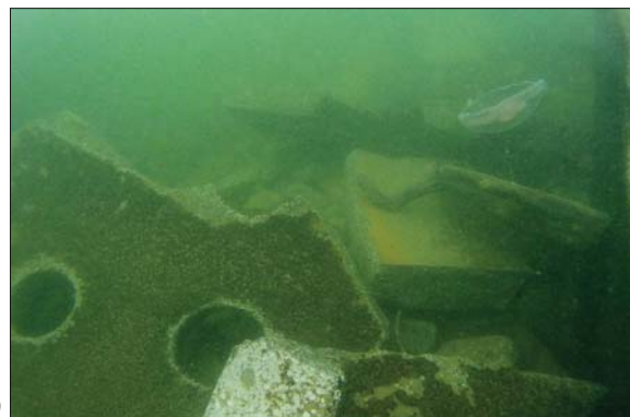
Fig. 9. Damaged elements under water
