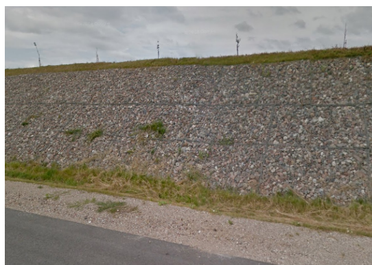
Figure 9. Frame construction of gabions at the Zambrów bypass
