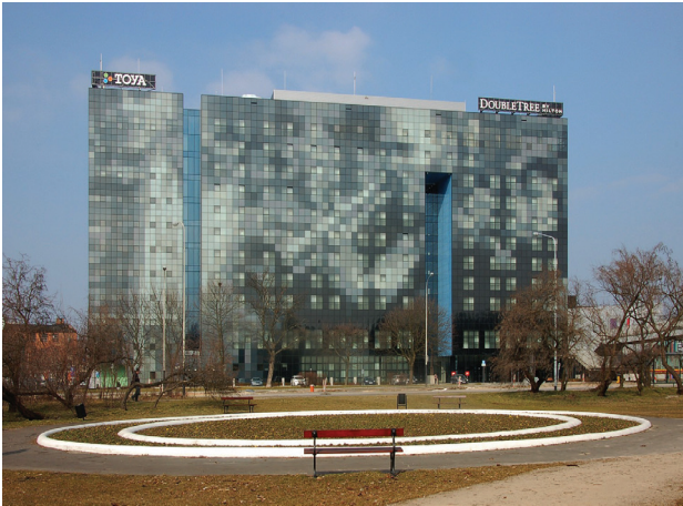
Il. 8. Hotel Double Tree by Hilton (studio Kuryłowicz & Associations 2013) (fot. Zeto, „Fotopolska-Eu”)
