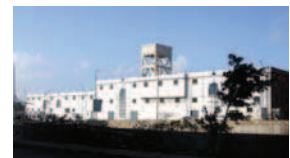
Fig. 14. Warehouse Bank Misr, facing the Canal
