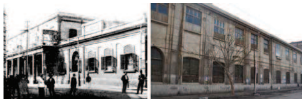
Fig. 4. Left: Old photo of the Bourse of Minet El-Bassal, designed by P. Avoscani 4 , and Right: new photo of the Bourse of Minet El-Bassal (Source: authors, 2012)
