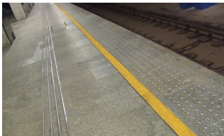
Figure 3. A physical components installed on the ground. The photo was taken with a smartphone Sony Xperia XA1 Ultra G3212 4 at the Warsaw Chopin Airport station. Own elaboration.
