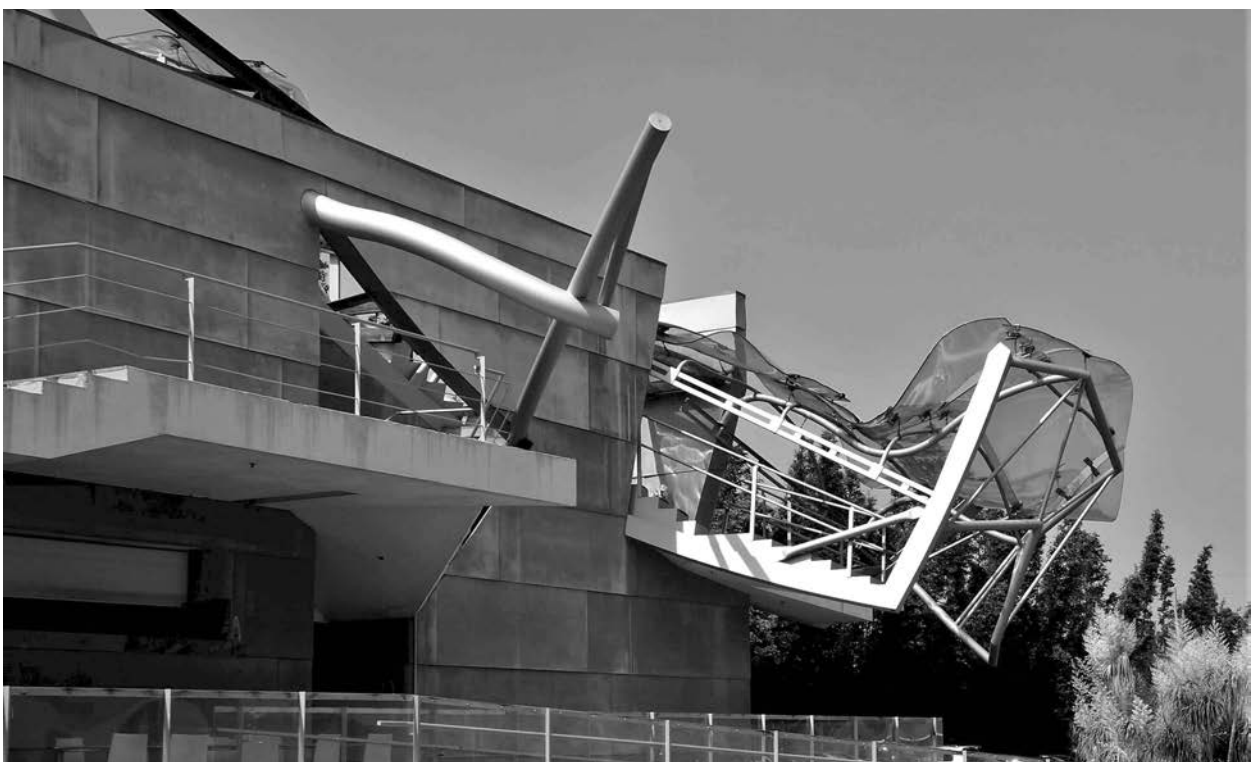
il. 8. Culver City, Umbrella, Eric Owen Moss (1999), fot. B. Malinowska-Petelenz
