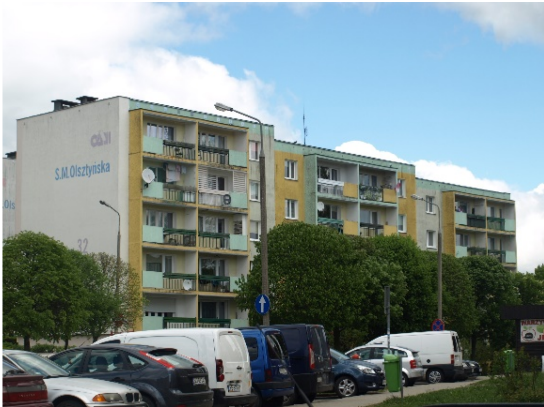
Figure 1. A residential building constructed in the Wk-70 large-panel system
