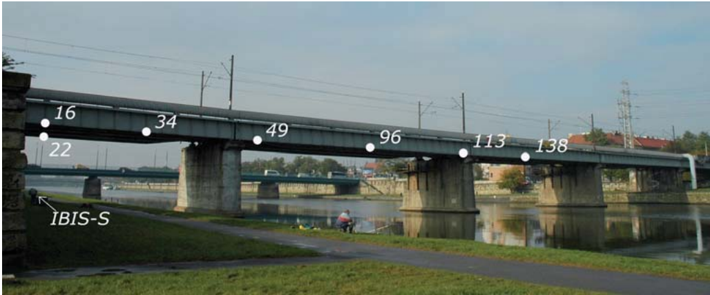
Fig. 7. View of the tested bridge with observed points marked
