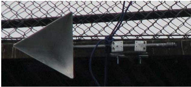
Fig. 6. Microwave reflector installed on an object
