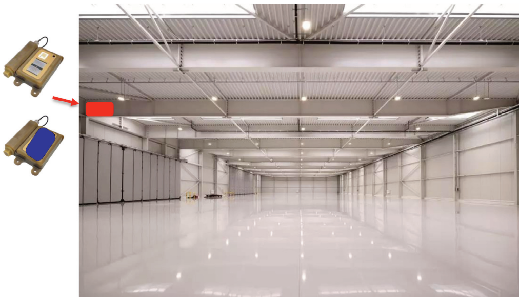
Figure 2. Example location of corrosion sensors on the hangar structure.
