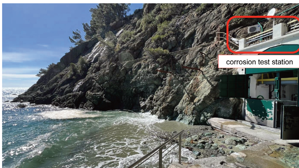
Figure 4. View of the corrosion test station in Bonassola.
