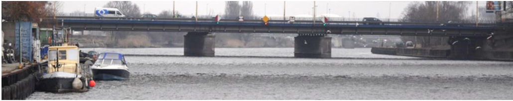
Figure 3. The Portowy (Harbour) Bridge (own picture)
