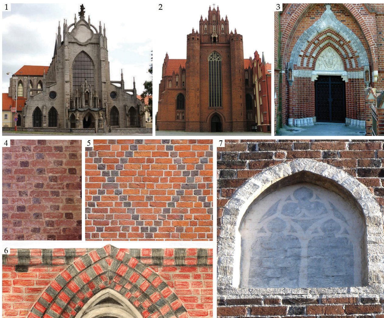
Fig. 7. Material color of the church façades in the 14 th century: 1 – Sedlec (photo by K. Charvátová), 2, 3, 5 – Pelplin, 4 – Lubiąż, 6 – polychrome in Henryków (photo and elaborated by E. Łuzyniecka), 7 – painting in Oliwa (photo by A. Piwek)
