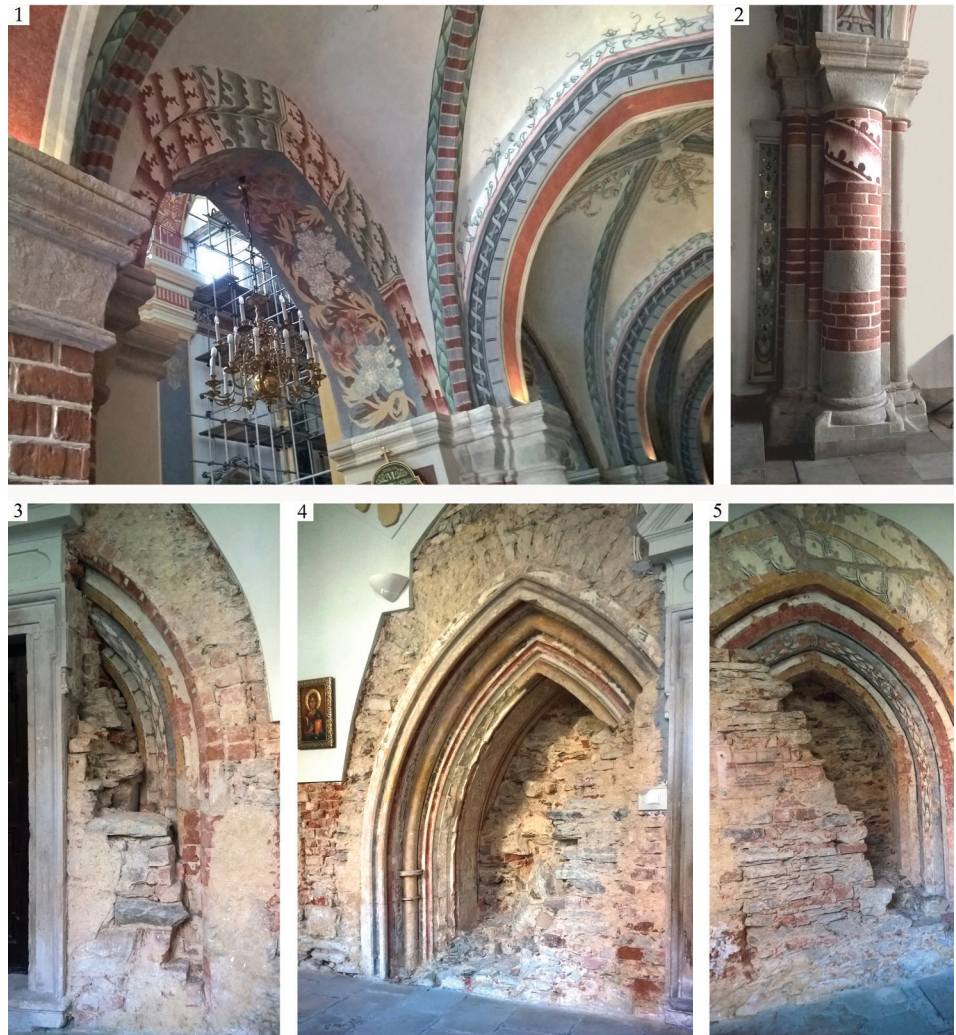
Fig. 9. Decorations of the interior. The monastery church in Mogiła: 1 – arcades and vaults, 2 – engaged column. The chapter house in Henryków: 3, 5 – relics of open works, 4 – portal (photo by E. Łuźniecka)
