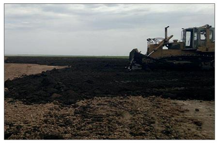
Figure 5. Applying a peat-sand mixture with a bulldozer
