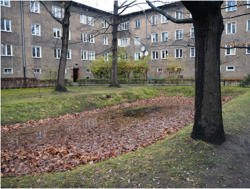
Fig. 2. Filled retention basin in Katowicka Street
