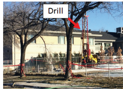
Fig. 1. Visible image of the shale gas leaks site as seen from the sensor location
