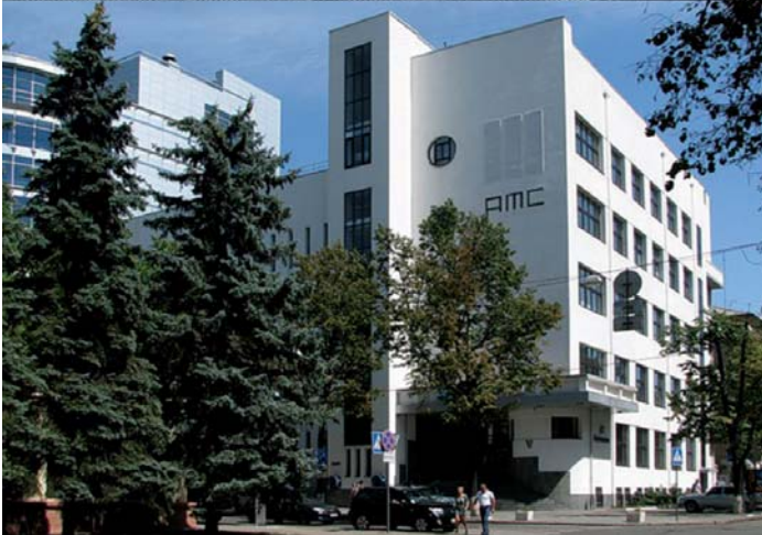
il. 8. Building of ATS. Pavel Frolov. 1930–1932
