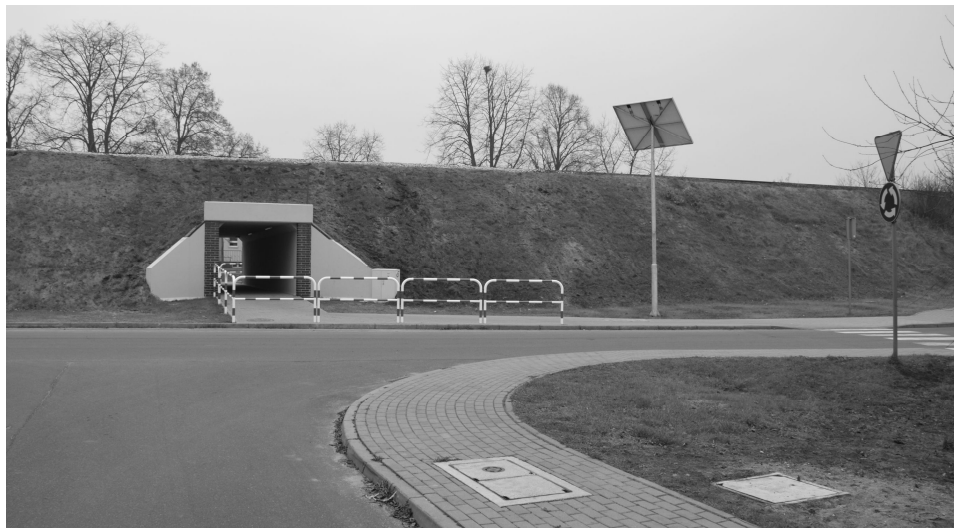
Fig. 6. View of a pedestrian crossing built under the railway embankment
