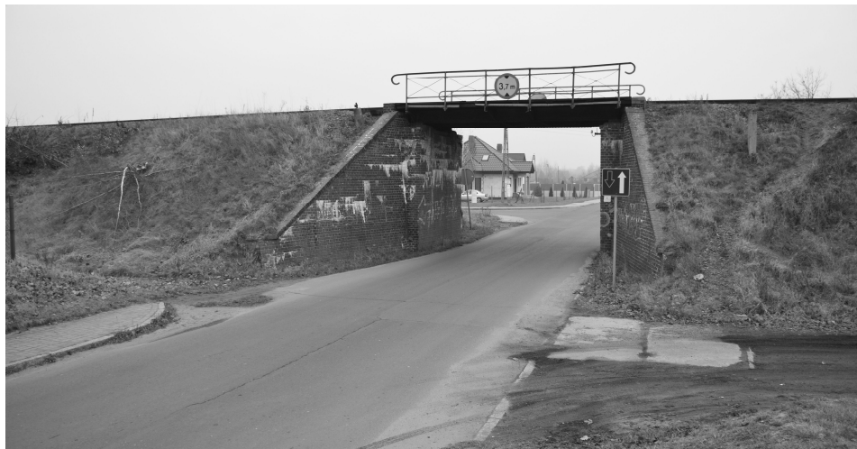
Fig. 3. View the railway viaduct over the street of General Walter
