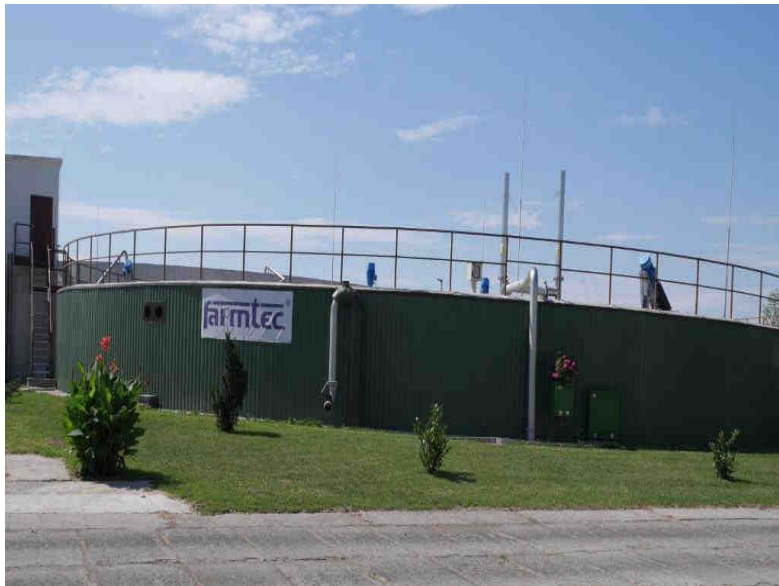
Fig. 1. Agricultural Biogas plant Agrodruzstvo Lhota pod Libčany, fermenter two-type “ring ring”
