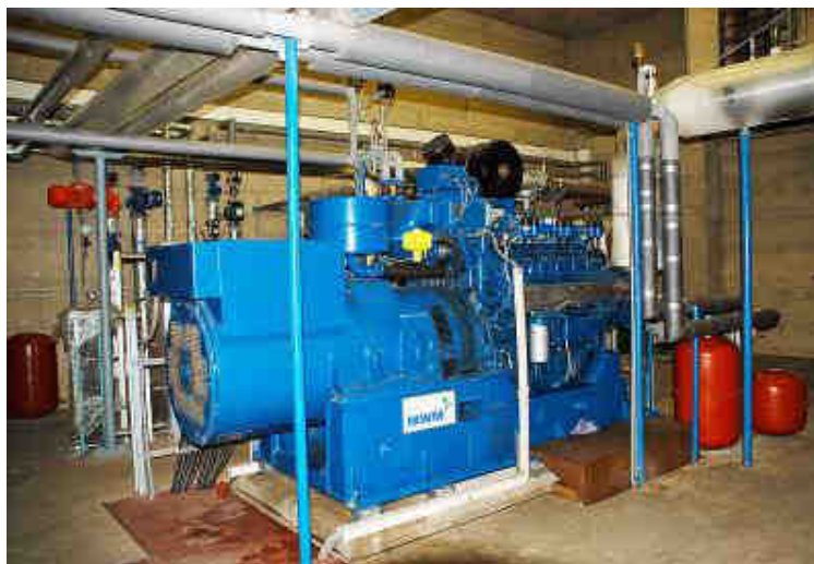
Fig. 2. Agricultural Biogas Cogeneration unit Agricultural Biogas plant Agrodruzstvo Lhota pod Libčany
