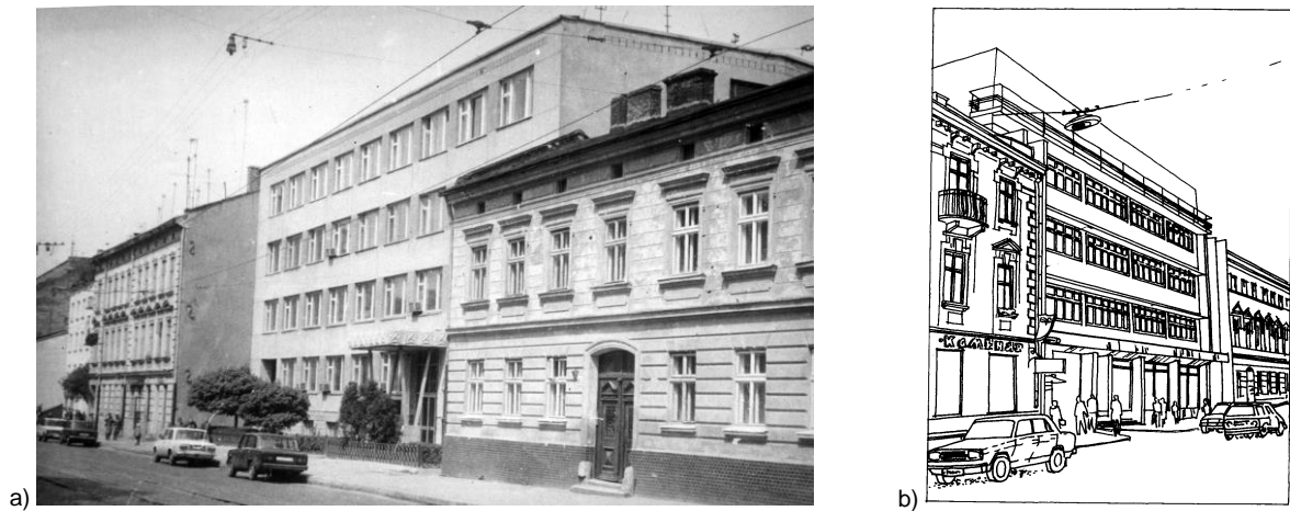
Fig.32. a) House of the project organization on Lychakivska Street. 1964. Source: Photo by B. Posatskyi, 1980.; b) Cosmetic salon on Ivan Franko Street. Source: Drawing from the photo of B. Posatskyi, 1980.
