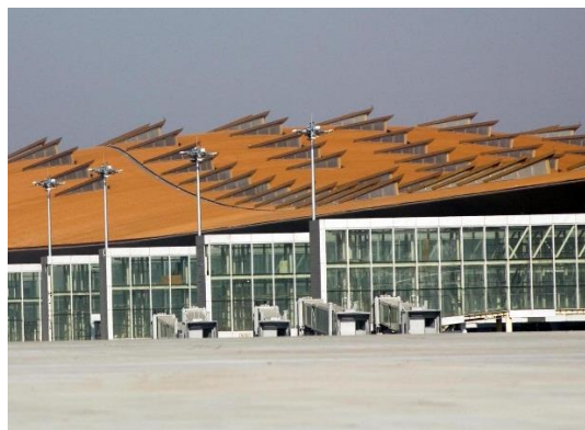
Fig. 2. Skylights on the roof. Source:[5]
