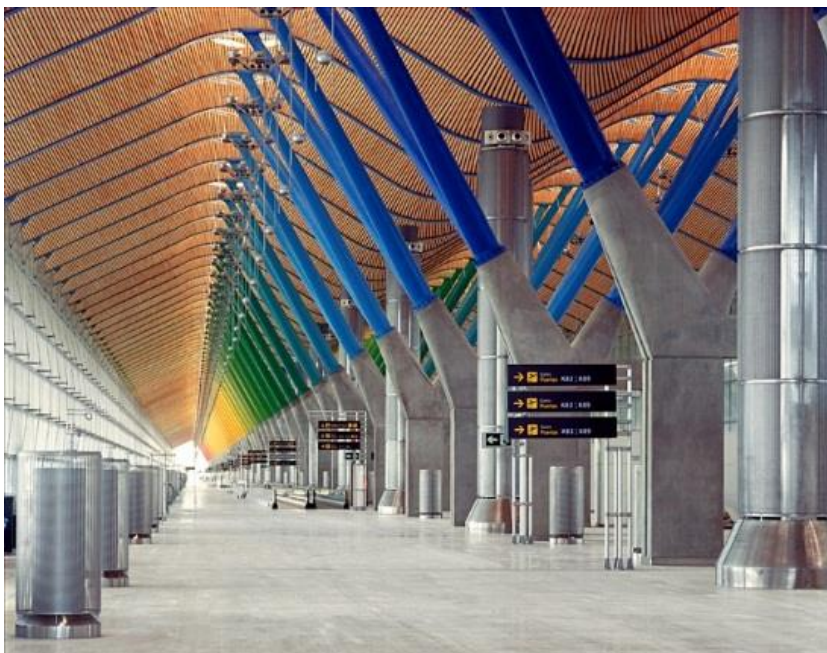
Fig. 9. The Y shape columns inside the airport. Source:[18]
