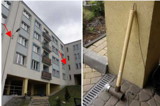
Fig. 1. The object under test, a four-storey building
