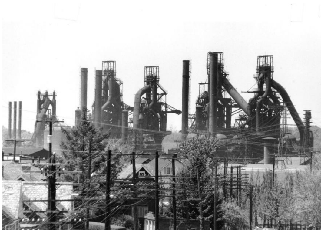
Fig. 1. A view of the former steel mill in Bethlehem. Source: [7]
