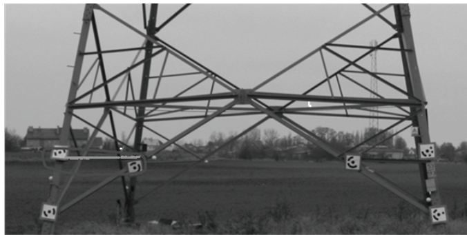
Fig. 7. The image of a piece of truss removed
