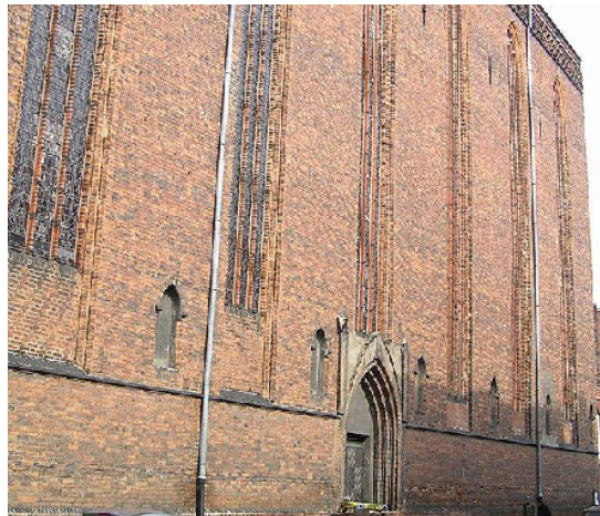
Fig. 3. A wall subjected to the measurements neighbouring Panny Marii Street.
