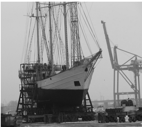
Figure 1. The ship at the repair post R4
