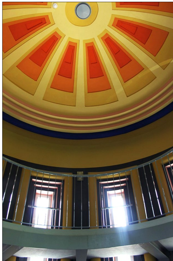
Fig. 6. The former "Hall of the Fallen" with its original architectural detail and color scheme restored, 2012; photo by I. Solisz
