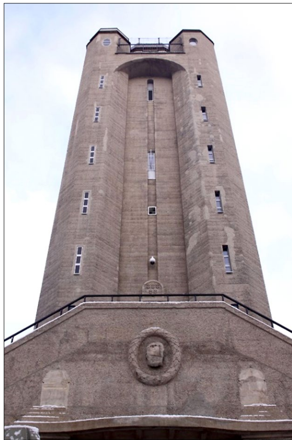
Fig. 10. View of the water tower from an unmanned aerial vehicle, 2019; photo by Ł. Bednarz
