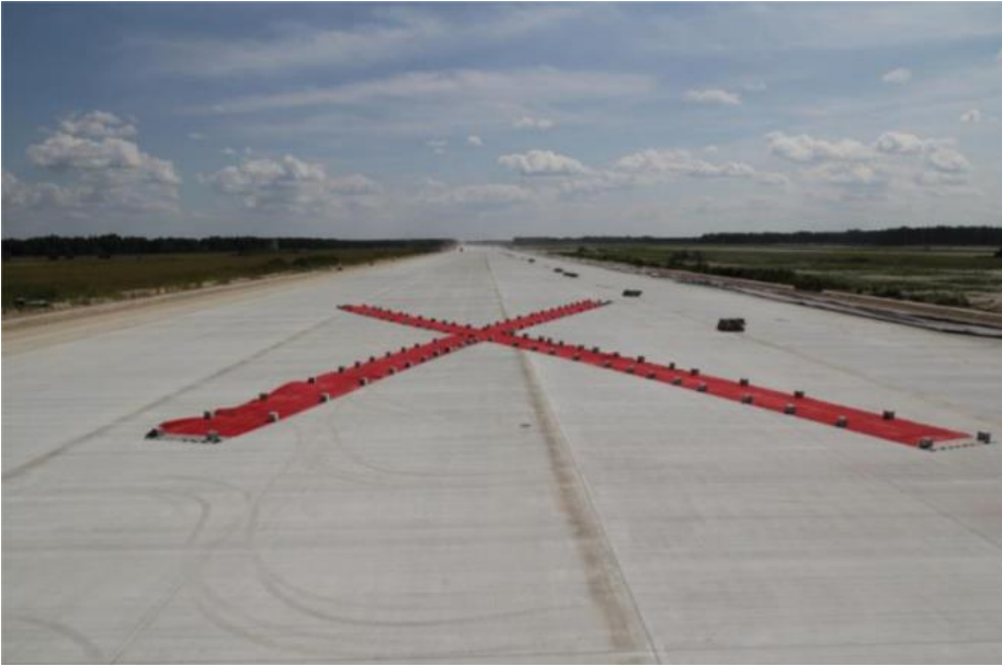
Figure 1. Marking in the middle of a closed runway under construction
