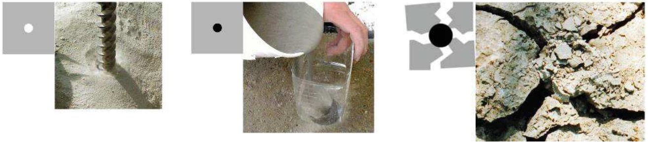
Fig. 9. Phases of the technological process of splitting rock solids with the use of expanding materials [22]
