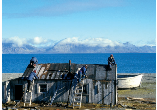
Fig. 17. The repair works on the building C (photo Janina Repelewska-Pękalowa 1986)
